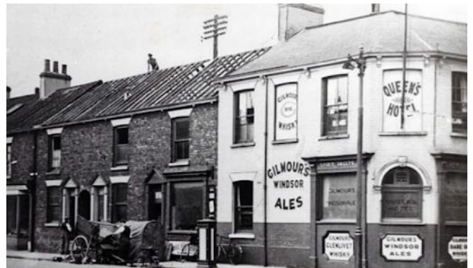
looking along Cambridge Street
